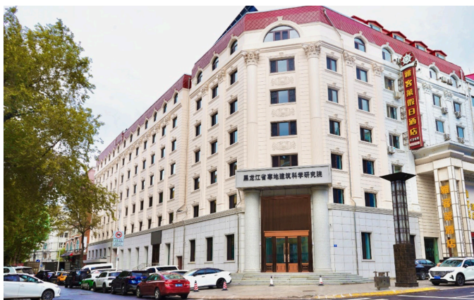
Figure 13: Outlook from street after renovation, source: Harbin DP
