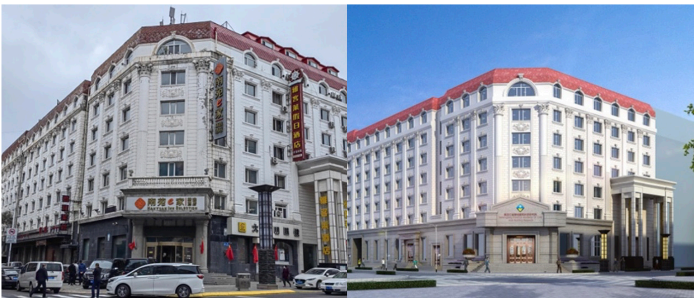
Figure 1: Photo before renovation and rendering after renovation. Source: Project Presentation 16.10.2023
