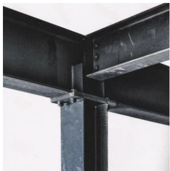
Steel structure 钢结构
