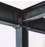
Steel structure 钢结构
