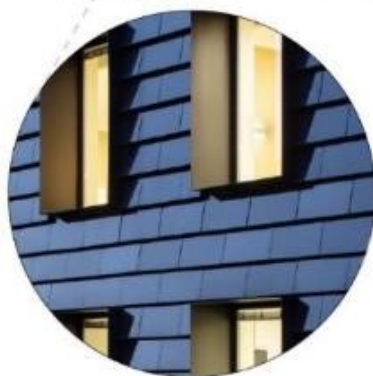
BIPV facade and roof
