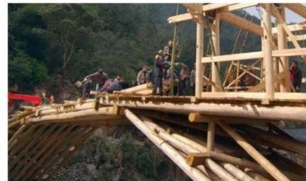
Arched Wooden bridge as pototype for large span structure
