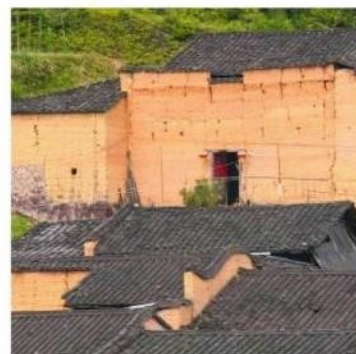
Rammed earth for Wall
