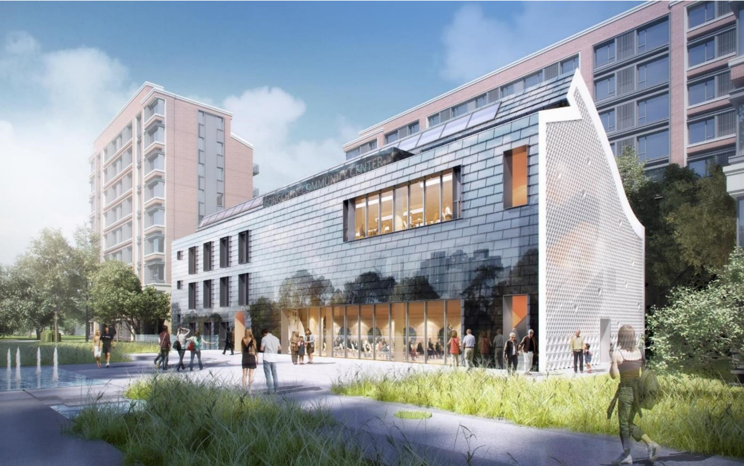
立面屋顶一体化：镜面光伏瓦与环境的互动 Photovoltaic panels on the south façade and south-side roof
