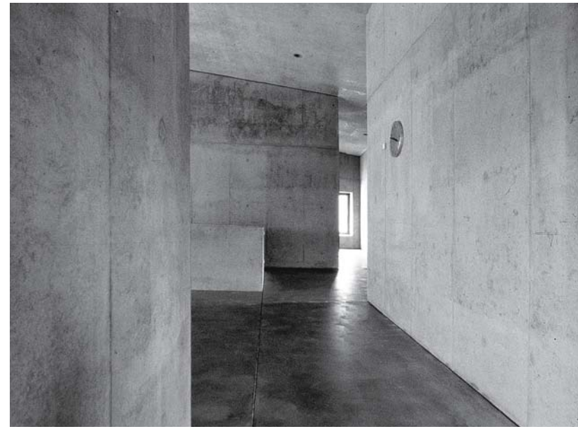
Fig. 140: Common area on 2nd floor
