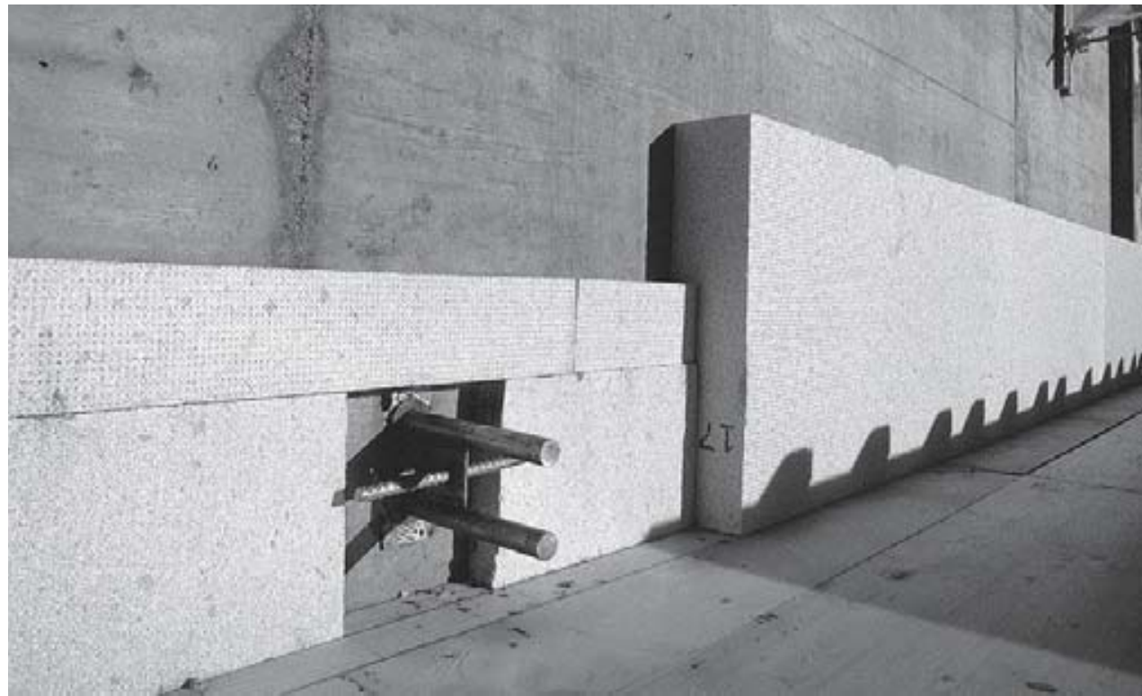
Fig. 134: The thickness of thermal insulation is reduced around the shear studs.
