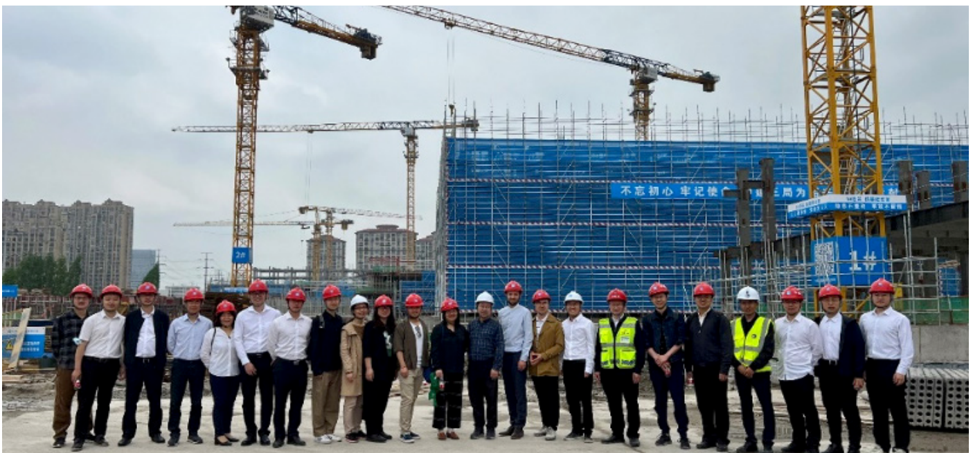
Figure 10: 2023.04.21 Project on-site visits and on-site technical exchange, Source: Sino-Swiss ZEB Project
