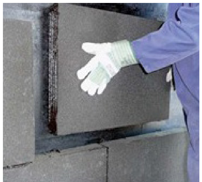
Figure 14: Foamglas, Source: Baufachzeitung Foam glass [Absolutely insensitive to moisture, durable/robust, medium to good insulation performance]
