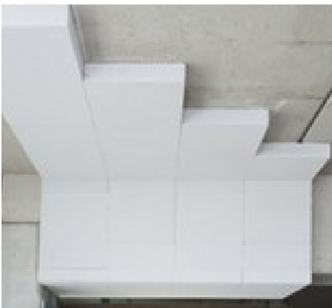
Figure 13: Calcium Silicate Insulation, Source: Xella Multipor Monolithic, mineral insulation (e.g. calcium silicate) [Diffusible & capillary-active, durable/robust, medium insulation performance]
