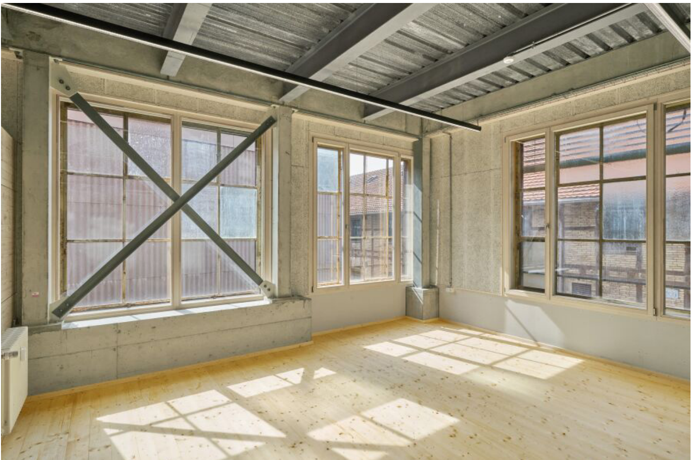
Figure 33: Example of surface-mounted electrical installation, Source: baubüro in situ «K118»
