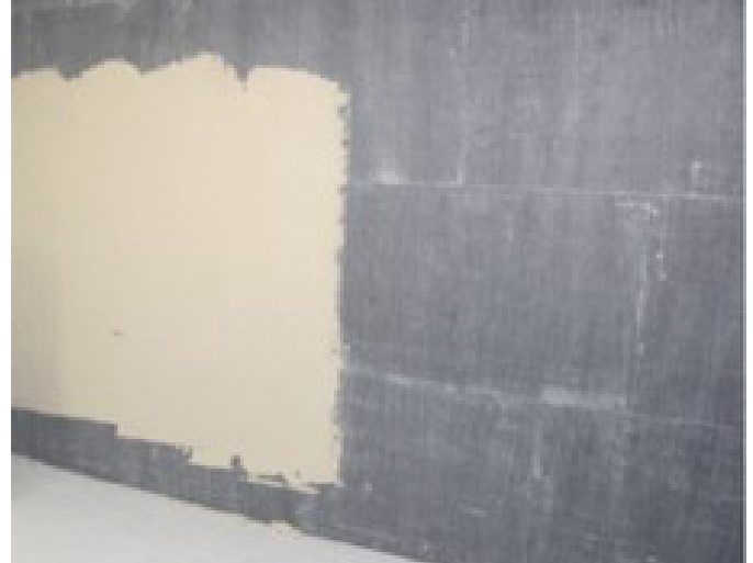
Figure 16: Aerogel fleece, Source: Agitec Spaceloft High-Performance Insulation (e.g. VIP, Aerogel, PIR)
