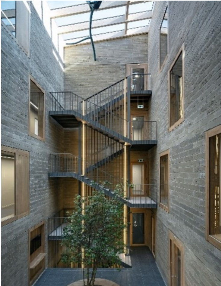
Figure 29: Claystone-walls as a climate-friendly alternative to mineral building materials in the atrium of the headquarters for the environmental authority, canton of Vaud. Source: Baud, Früh architects
