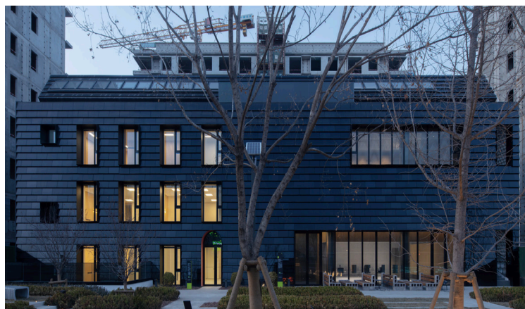
Figure 15: Yinyue Zero-Carbon Building, Fangshan District, Beijing (Source: Gallery of Architecture for Sustainable Development Goals)
