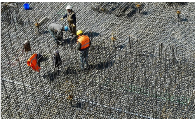
Figure 4: Construction side (Source: pixaba)
