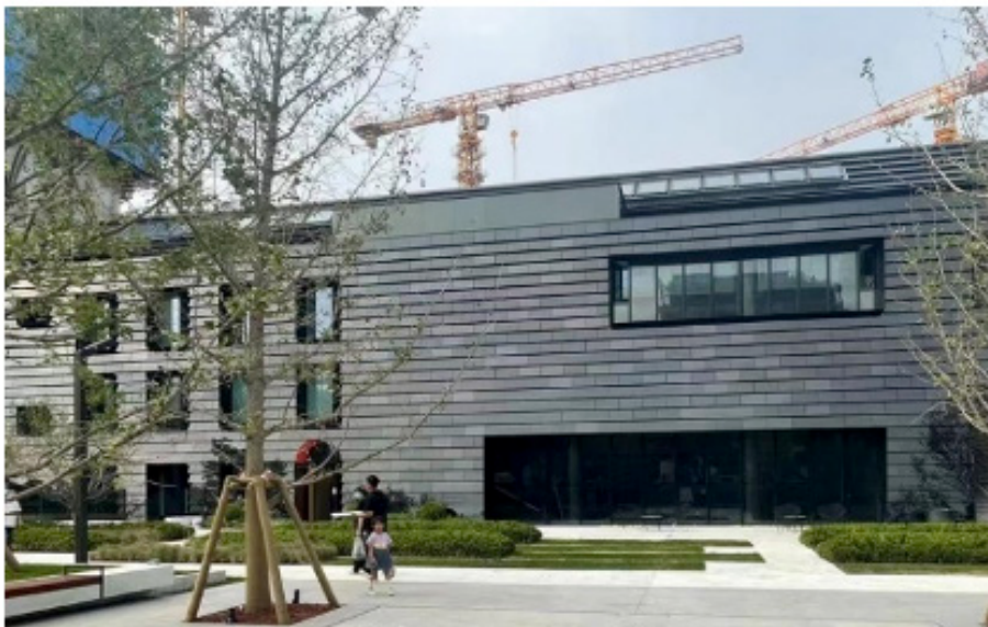
Figure 15. Mock-Up of BIPV and the built BIPV, Source: Project Presentation 17.11.022 and Site Visit 19.10.2023 ©SUP Atelier
