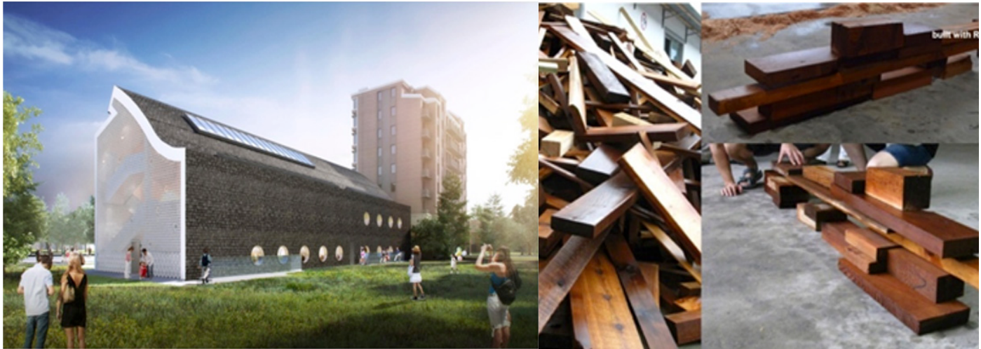
Figure 6. Recycled wood on north façade was planned, but unfortunately not implemented due to quality control concerns. Instead, new wood was montaged on façade. Source: Project Presentation 17.11.2022 ©SUP Atelier
