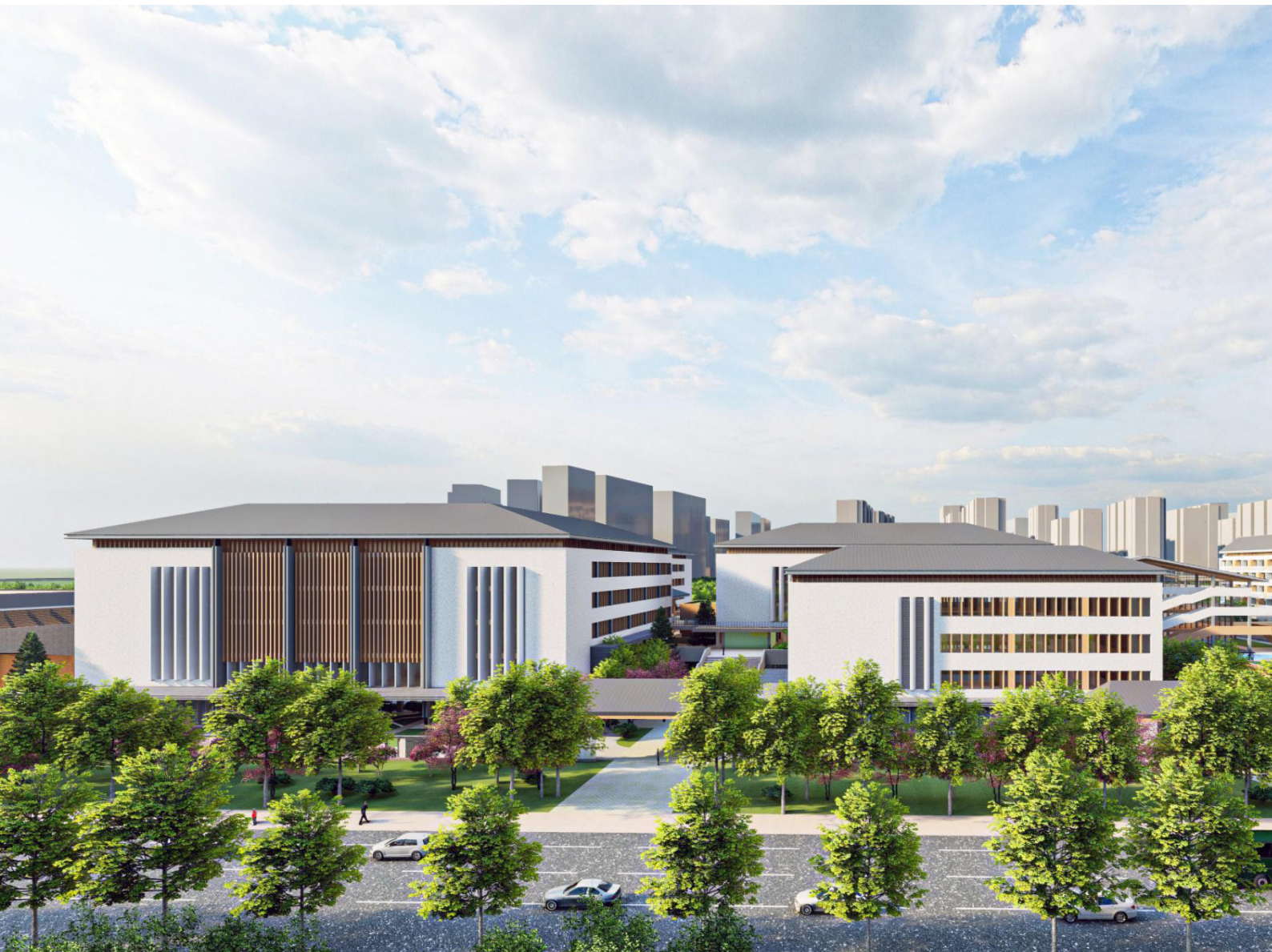
Image: ZEB China Demonstration project. Training building, Long Shan Shu Yuan Middle School, Shaoxing, Zhejiang Province. Courtesy of Shaoxing Future Community Development and Construction Co.
