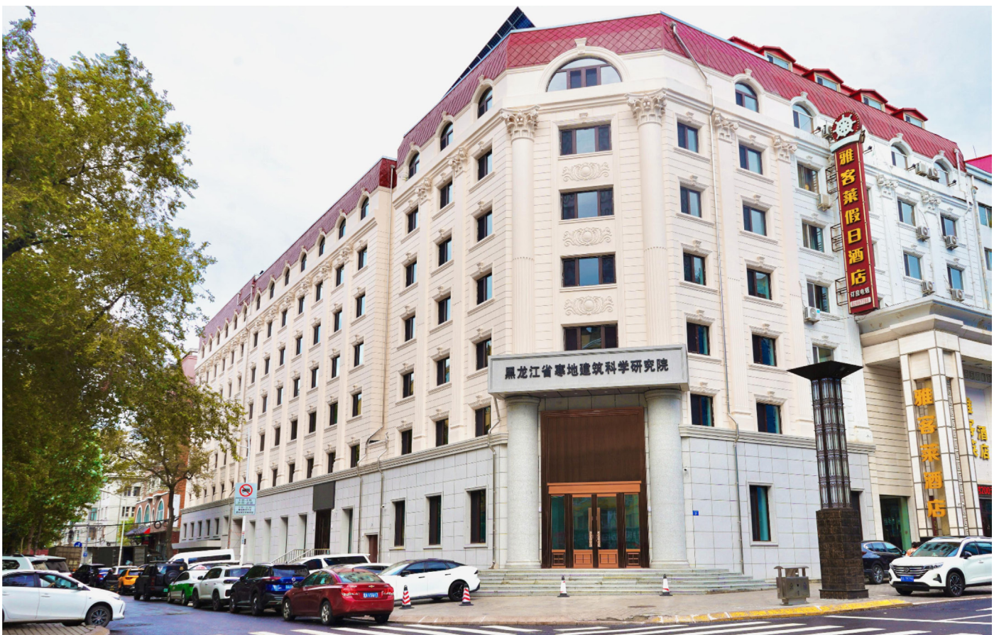
Figure 4: project façade after renovation. Source: DP Harbin.
