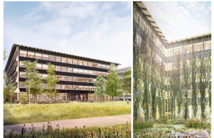
Figure 31: Hortus, Allschwil near Basel, movable, horizontal PV modules on the outer façade (left) produce electricity and serve as sun protection, in the inner courtyard (right) the façade was greened (© Herzog & de Meuron)
