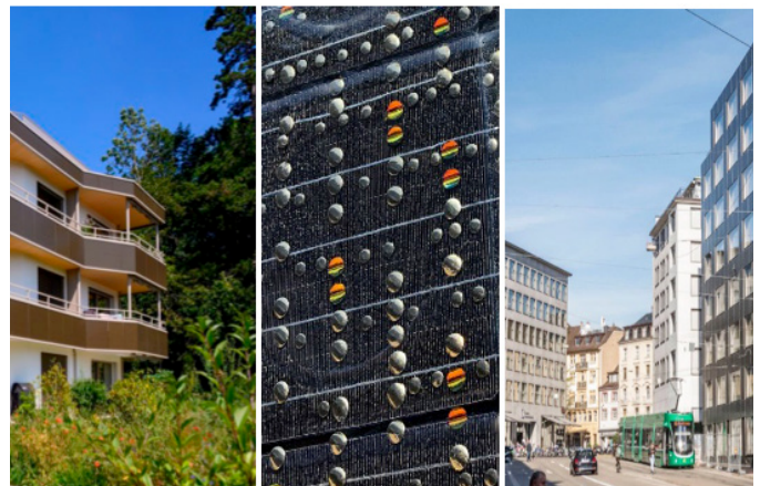
Figure 32: left: Residential building in Zurich, Höngg, opaque PV modules design the façade of the residential building (© Kämpfen Zinke + Partner AG); middle & right: Office for Environment and Energy in Basel, customized PV panels give the building its expression (© AUE)
