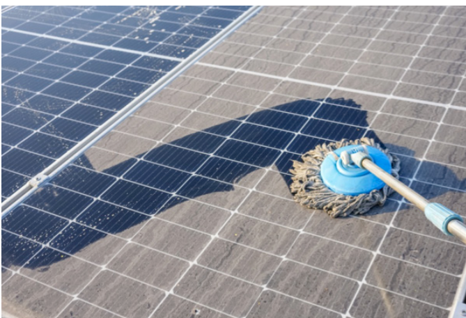
Figure 6: Pollution can reduce the electricity output, regular cleaning is recommended © AdobeStock
