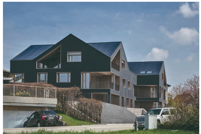
Figure 1: MFH Brütten © 3S Swiss Solat Solution
