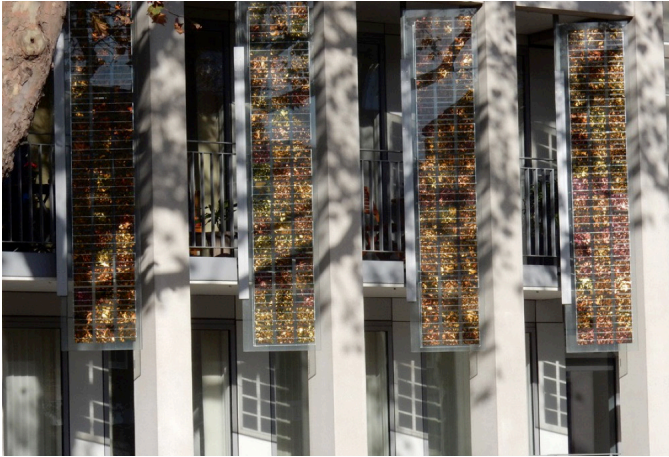
图5 应避免光伏组件受到阴影的影响降低发电效率 © Kingsgate House, London / P. Bonomo
