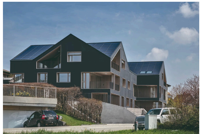
图1 MFH Brütten © 3S Swiss Solat Solution
