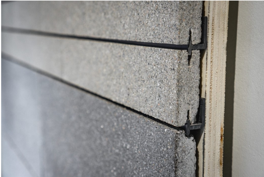
Figure 46: A detail image of the anchoring system of the Beyond Wall System © BEYOND WALL SYSTEM
