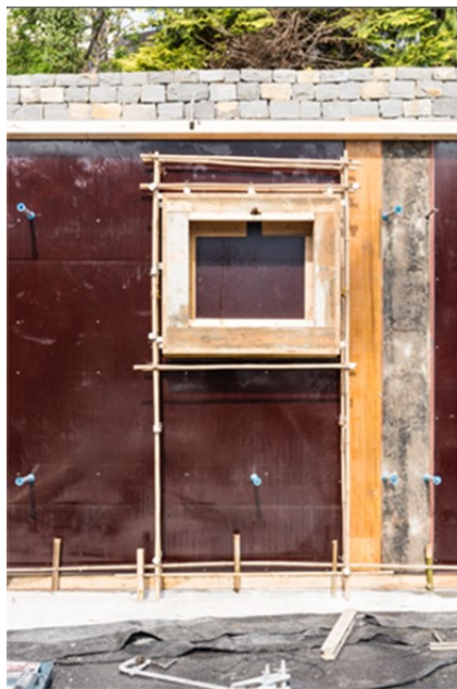
Figure 34: CONSTRUCTION PHASE OF THE UNDERGROUND LEVEL OF THE HOUSE K IN ALPNACH, SWITZERLAND. ©RASMUS NORLANDER
