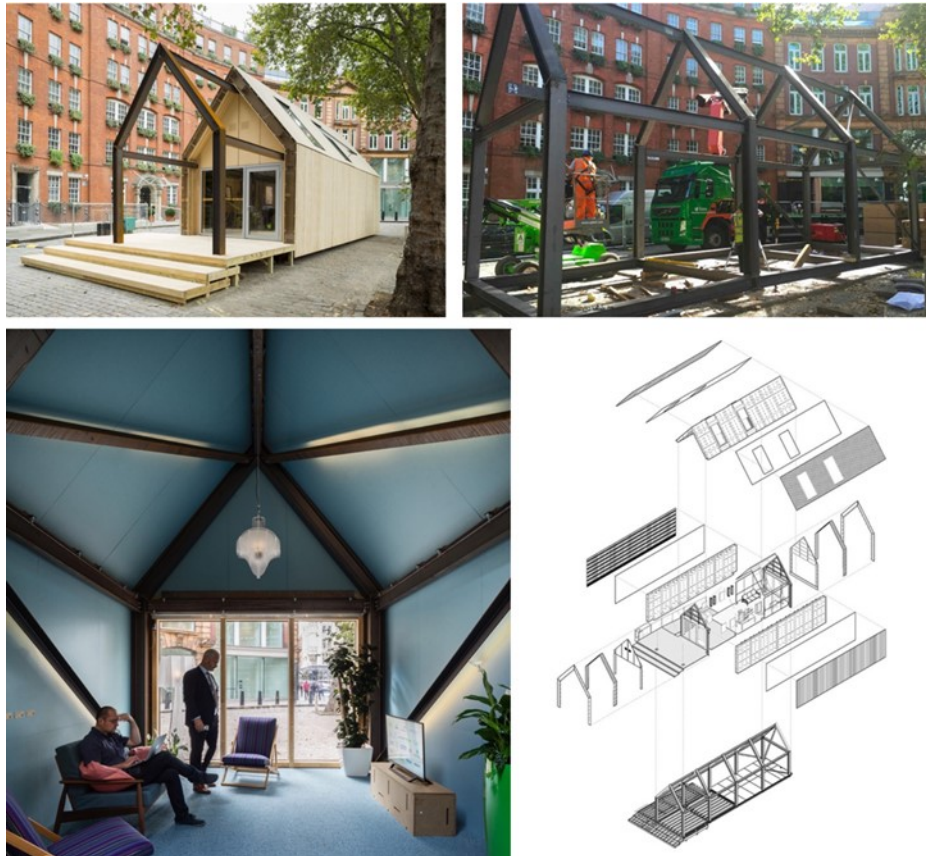
Figure 20: FROM LEFT TO RIGHT: AN INSTALLATION CREATED OUTSIDE THE BUILDING CENTRE FOR THE LONDON DESIGN FESTIVAL 2016. THE STEEL STRUCTURE OF THE CIRCULAR BUILDING. THE INTERIOR SPACE OF THE CIRCULAR BUILDING. EXPLODED AXONOMETRIC VIEW OF THE STRUCTURE AND ELEMENTS OF THE CIRCULAR BUILDING. ©ARUP
