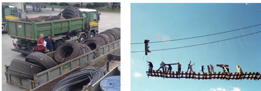
Figure 19: TRANSFER OF CABLES AND THEIR USE IN THE CONSTRUCTION OF THE BRIDGE. ©VANDERWALM
