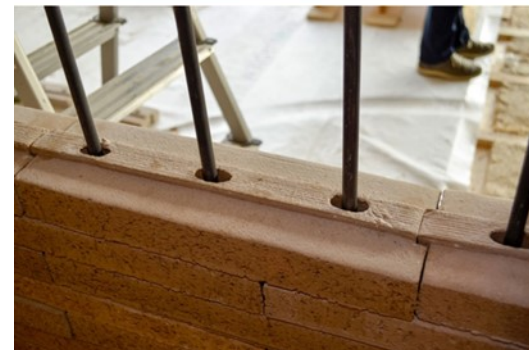
Figure 45: Built example of a movable wall partition with recycled Brics Stonecycling © BEYOND WALL SYSTEM
