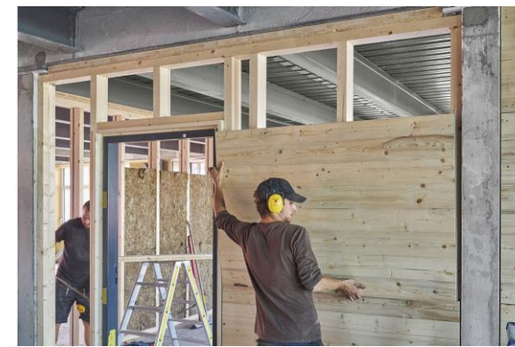
Suggestion 1: Wooden Stud construction with coupled wooden frames 建议一：采用双联木框架的木螺栓墙体结构
