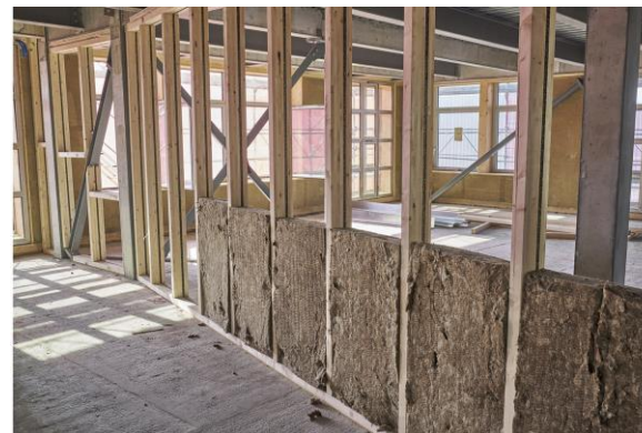
Suggestion 1: Wooden Stud construction with coupled wooden frames 建议一：采用双联木框架的木螺栓墙体结构
