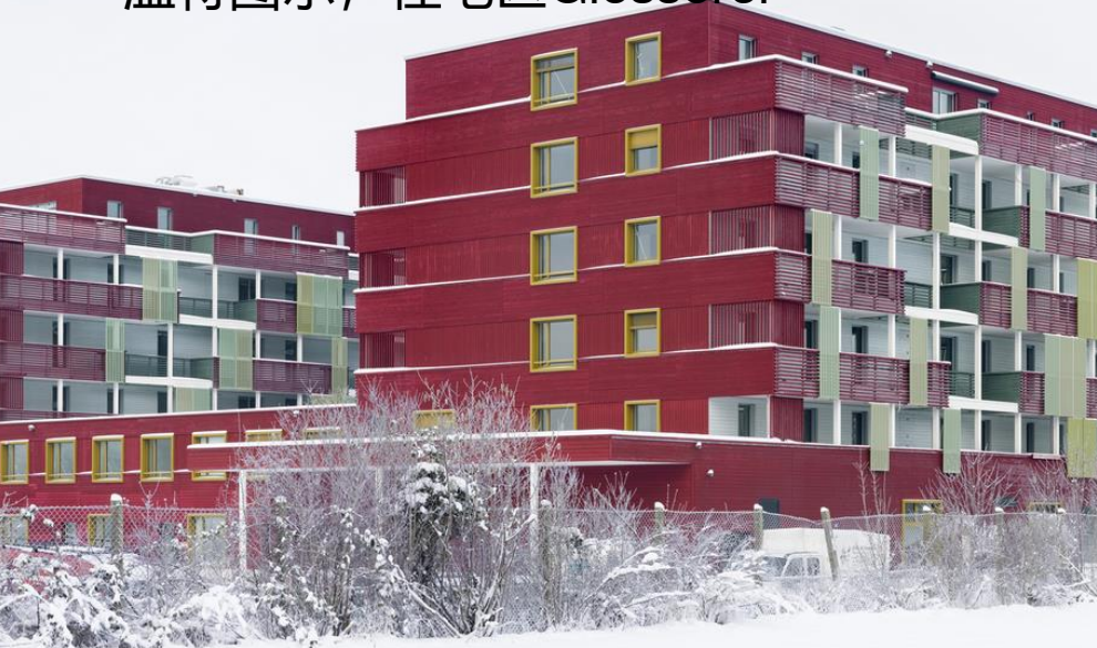
Winterthur, Residential Area Giesserei 温特图尔, 住宅区Giesserei
