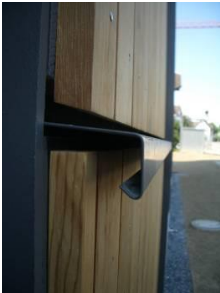
Fire stop barrier on timber façade 木制外墙的防火隔离带
