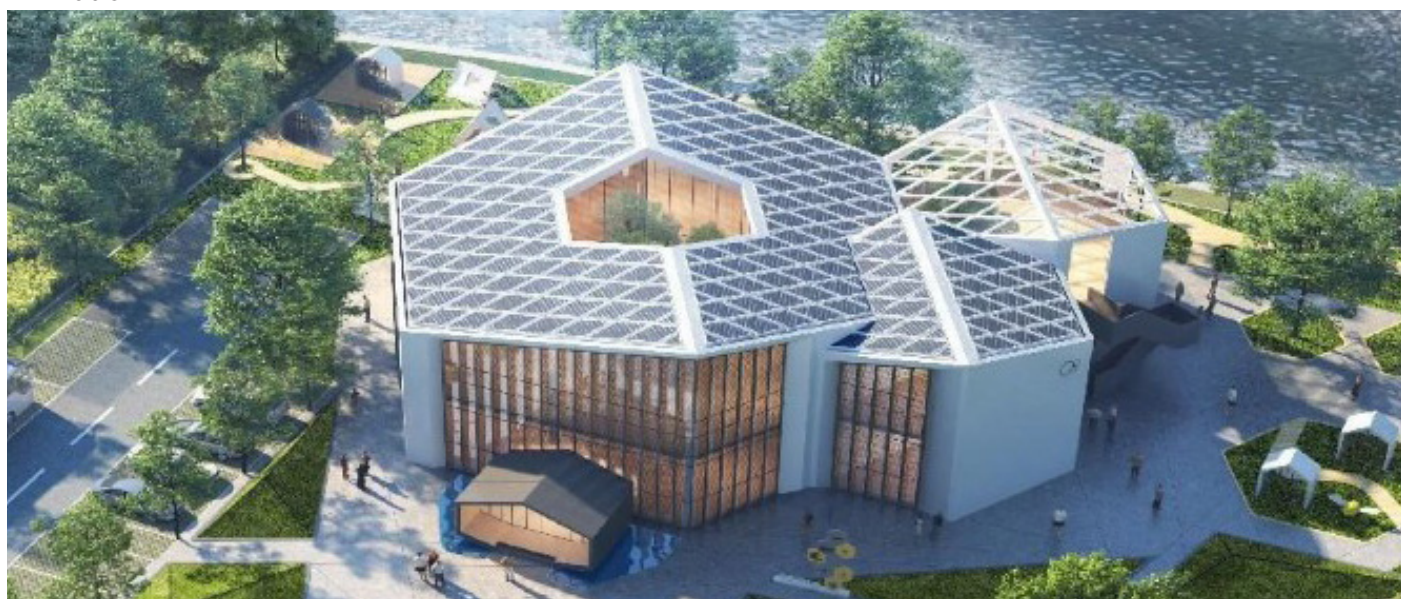
Image. Chinese Honeybee Museum, Liuba County, Hanzhong City, Shaanxi Province (Beijing Demo Project of Sino-Swiss ZEB co-operation project)
