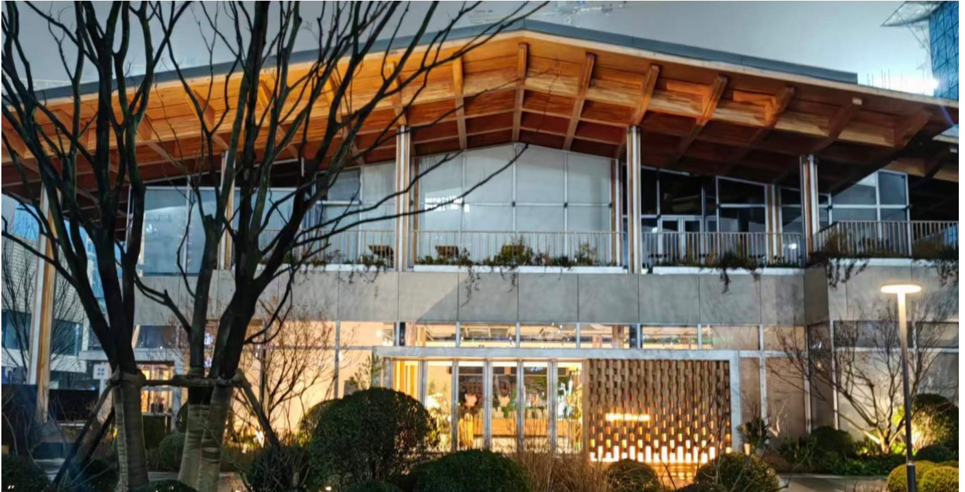
Image. Market Building and Exhibition Building Jiading, Shanghai (Beijing Demo Project of Sino-Swiss ZEB cooperation project)
