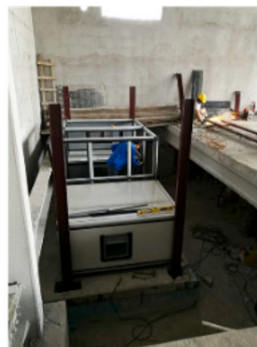
Figure 11. Zero carbon strategy – Active technology “fresh air heat recovery”, Beijing Demo Project of Sino-Swiss ZEB cooperation project - Gongchen Community Center of Fangshan District in Beijing. Graphics created by SUP and ZEB consulting Team of CABR.
