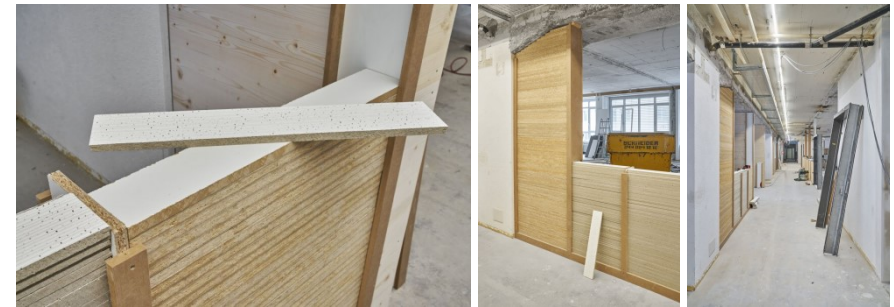
Figure12 Construction of Transa interior wall © baubüro in situ/ Martin Zeller
