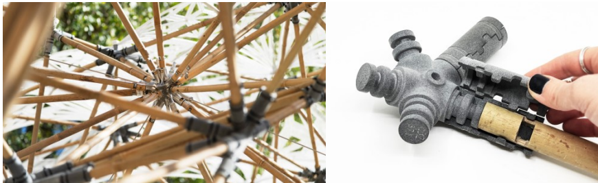
Figure14 Connection nodes in Digital Bamboo ©dbt/ Marirena Kladeftira
