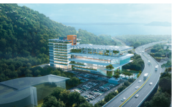
Shenzhen Nanshan Energy Ecological Park Zero Carbon World, Shenzhen
