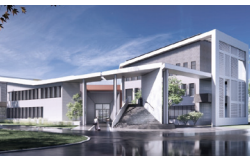
Taixing Development Zone Waterworks Phase II, Taixing, Jiangsu Province
