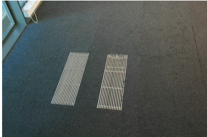
Figure 14: Floor-Level Air Supply HVAC Unit
