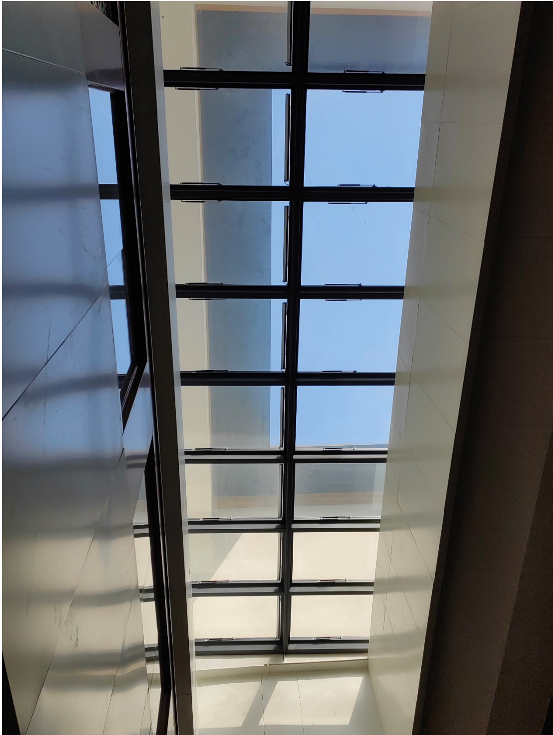
Figure 8 Operable Skylight in the Building Atrium
