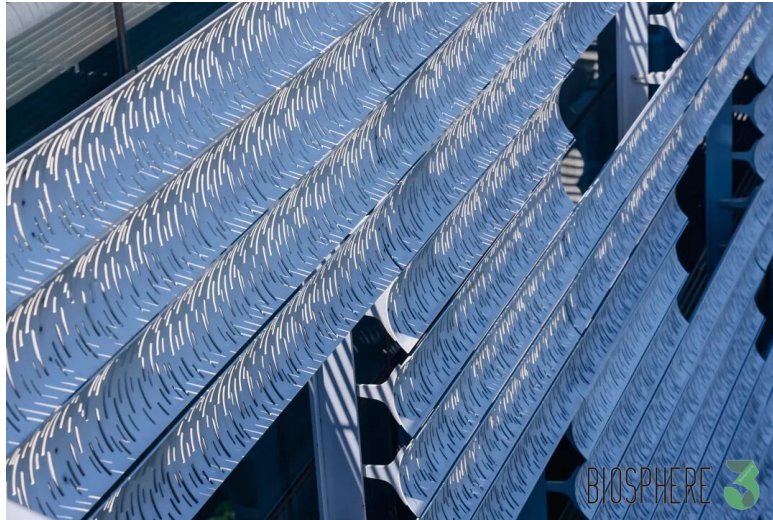
Figure 13: Building Exterior with Aluminum Panel Shading 7
