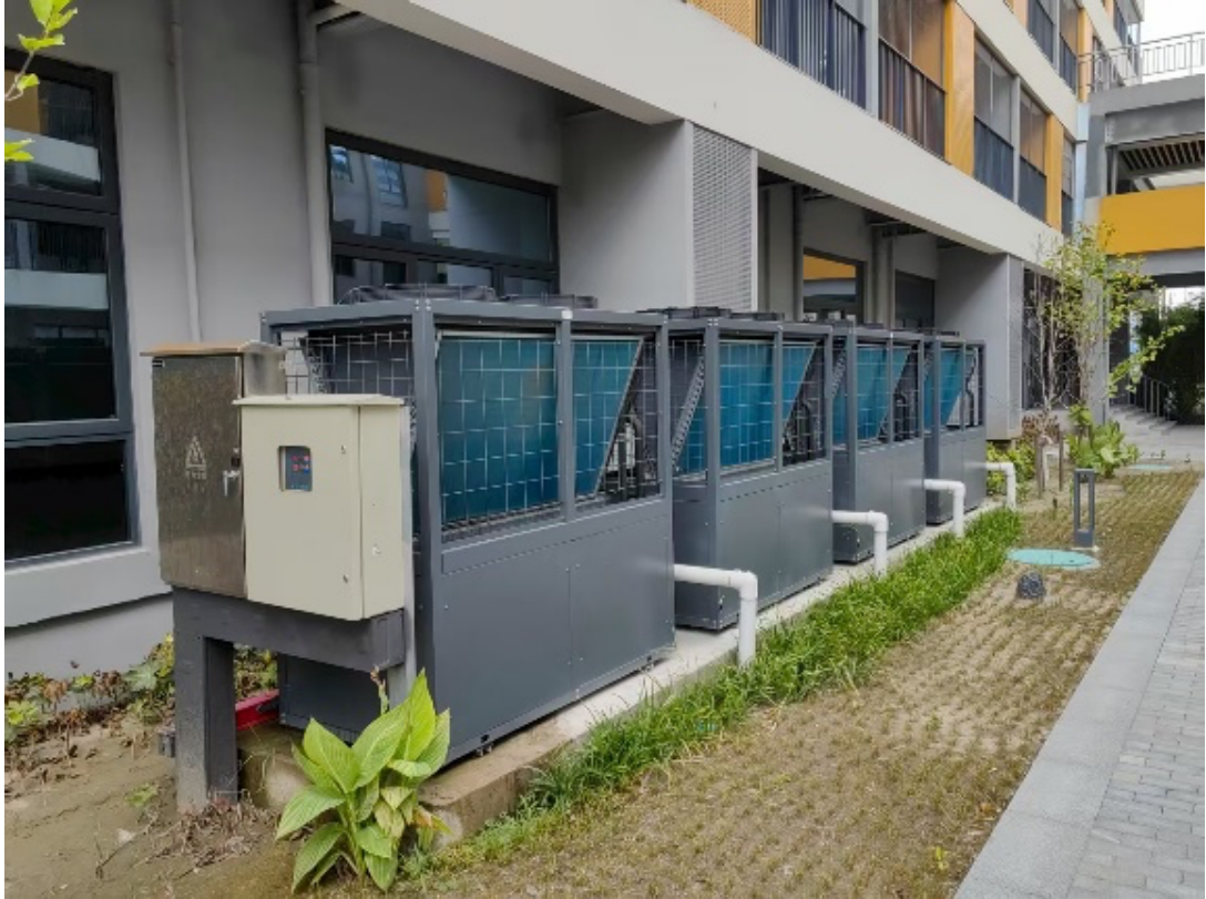
Figure 1 Air-Source Heat Pump Unit Located Below the Dormitory Building
